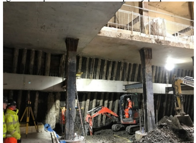
Figure 8 B3 permanent and T2 temporary props
