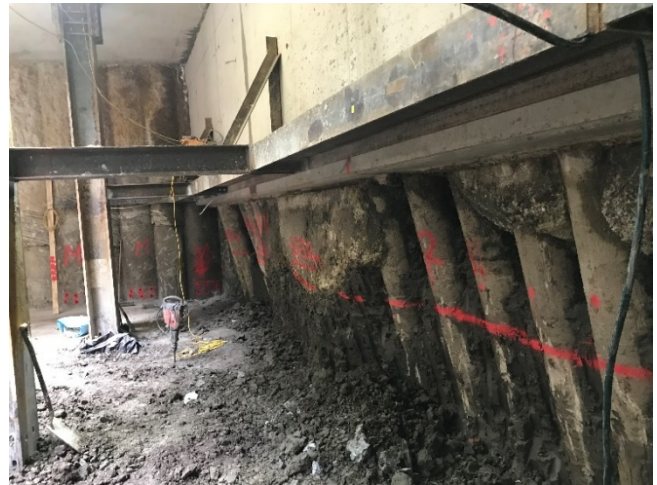
Figure 7 Variability of the D-wall toe level
